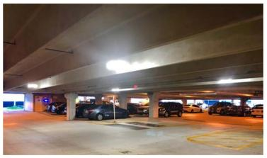
Technical and economic analysis for the new luminaires of 66-Watt CREE IG Series LED Parking Garage Luminaire for the NSU HPD Parking Garage in replacement of the existing 150-Watt High-Pressure Sodium Lamps. The Nova Southeastern University, Davie, Florida – U.S.A.
